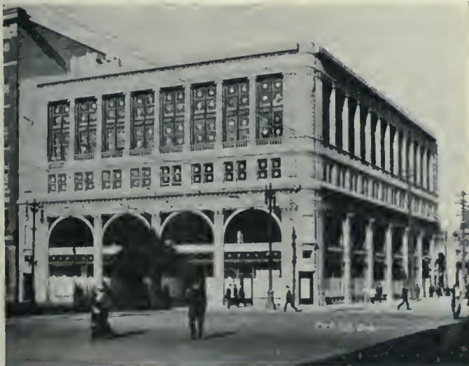
Paris Building, Winnipeg—completed.
